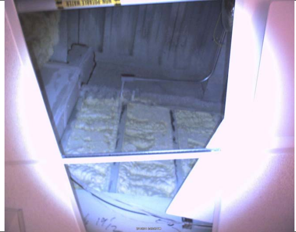
Figure 13 Another location of the showing the air leak at the top of the wall demising wall between garage and conditioned space. The bright vertical lines are infrared reflecting off the shiny steel studs.
