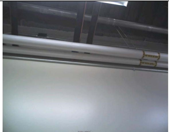
Figure 15 Air leakage around pipes penetrating the wall between the garage and the conditioned space. There are a number of locations where ducts, conduit and pipe penetrate the garage walls that must be
