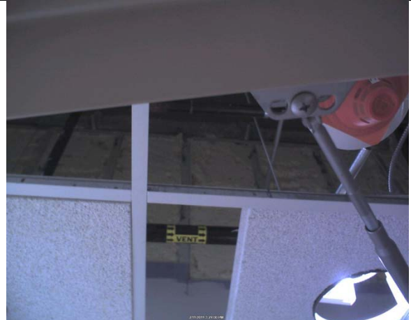
Figure 14 Another location showing air leakage through the fire lagging at the top of the garage demising wall.
